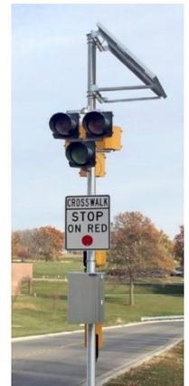
The Pedestrian Hybrid Beacon (PHB) provides more flexibility and options for the State Highway Administration at problematic pedestrian crossings. When a pedestrian wishes to cross the street, they can activate the signal and cars are required to stop.
